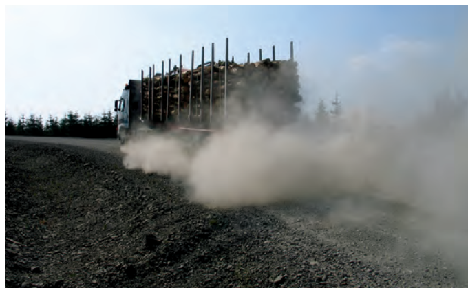
Figure 8 Blow-away of dry road material.
