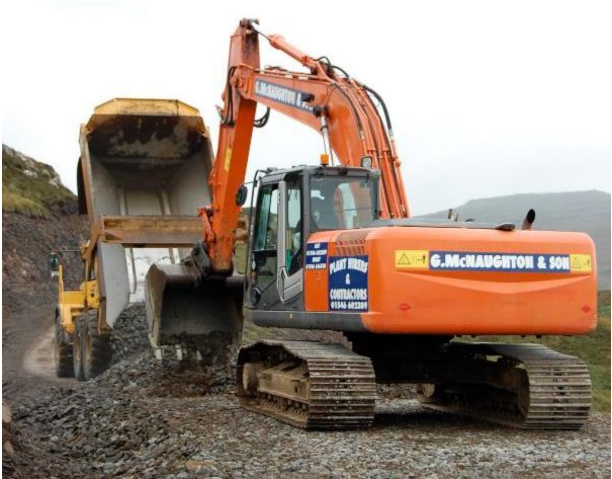
Figure 11 Forest road construction Photo Confor
