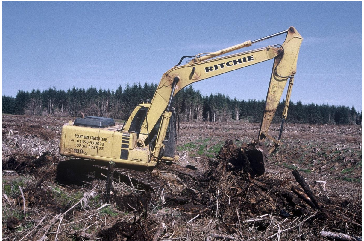
Figure 4 An excavator creating planting sites for restocking a harvested plantation, Photo Forestry Commission Crown Copyright
