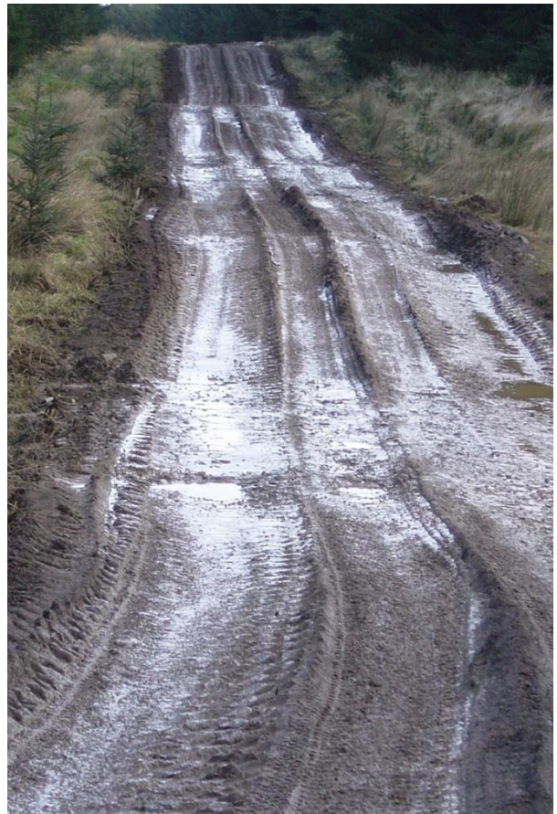
Illustration 1: Soft forest road trafficked by JST tractor would normally be impassable
