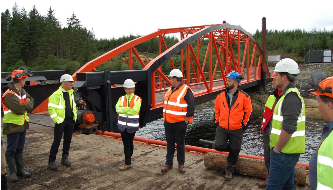
Figure 5 View of linkspan bridge from barge
